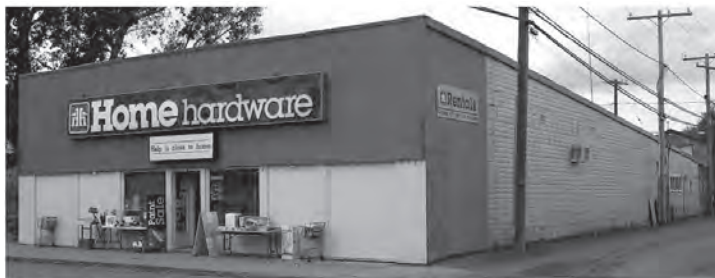
Buildings as it looks today
