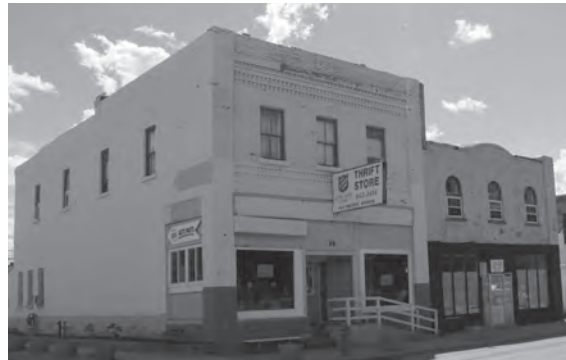
Buildings as it looks today
