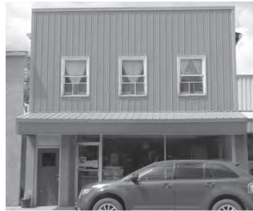
Buildings as it looks today
