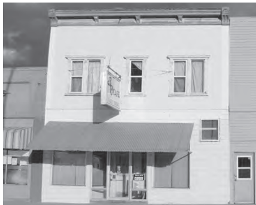
Buildings as it looks today
